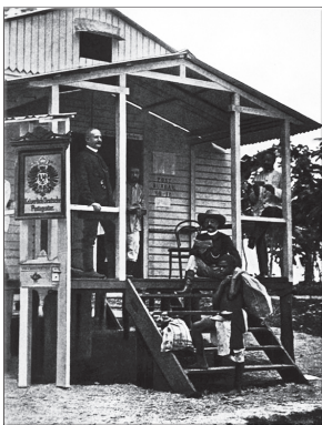
Post Office, Finschhafen, 1888
